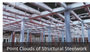
Point Clouds of Structural Steelwork
